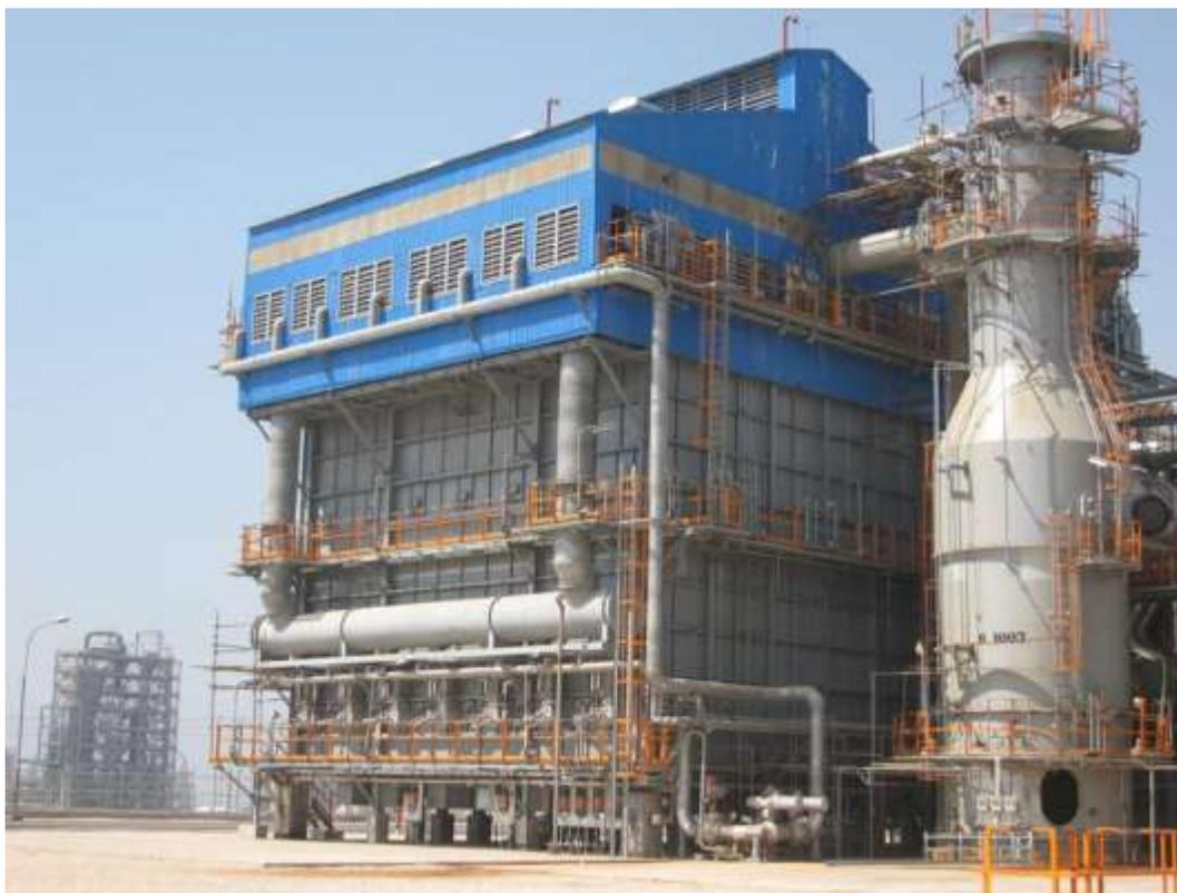
**Figure 21 - Primary and Secondary Reformer:** *Source: FEPCO.org*
